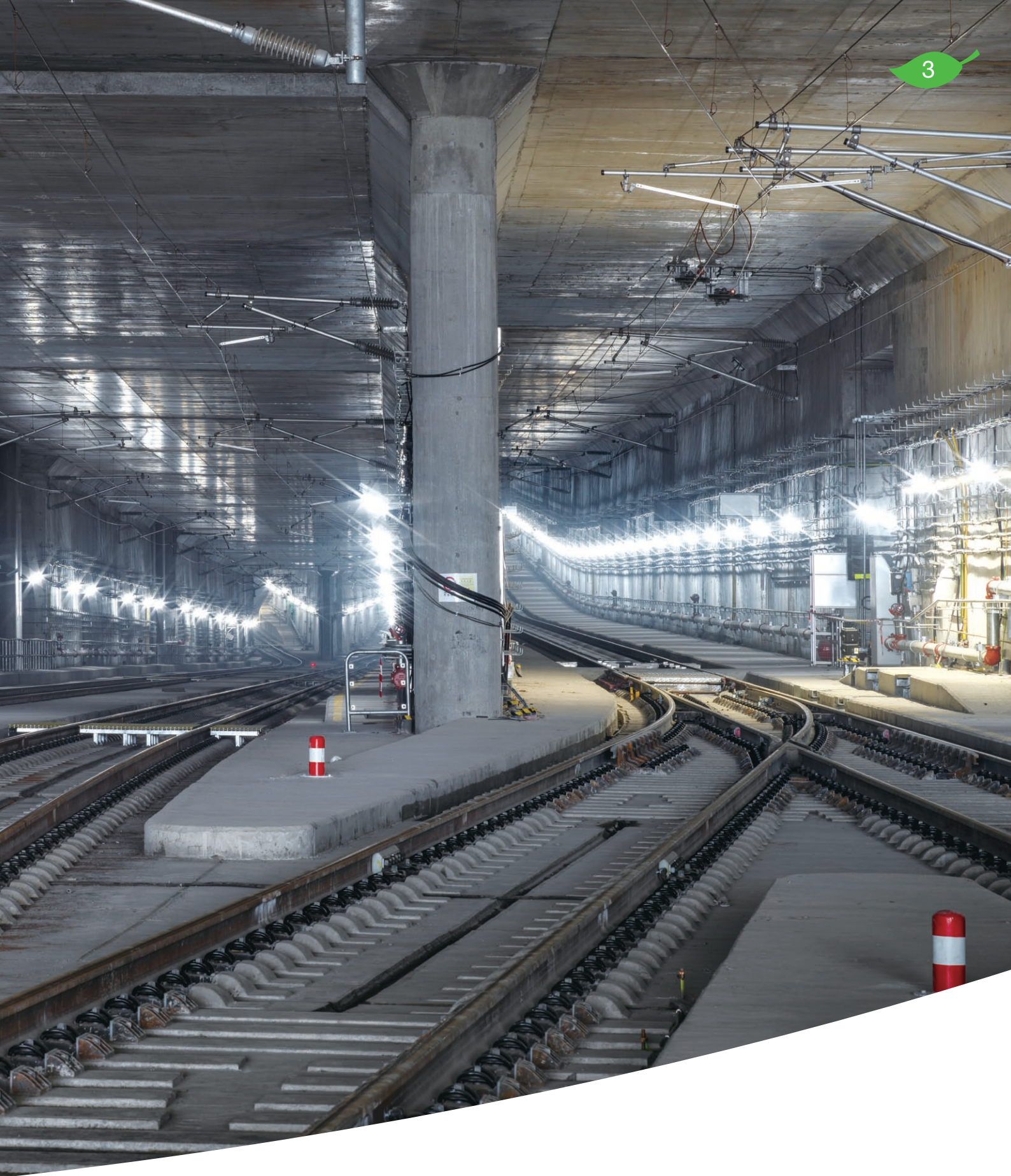
3 MTR Contract No. 830 – Guangzhou-Shenzhen-Hong Kong Express Rail Link (Hong Kong Section): Trackwork and Overhead Line System 港鐵合約編號830－廣深港高速鐵路(香港段)：軌道及接觸網系統
